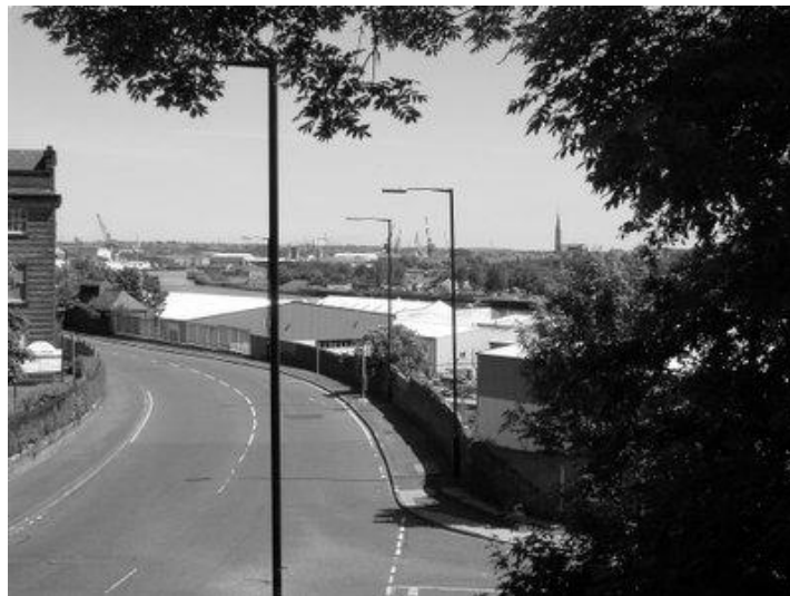
Figure 1 Road separating Walker community and riverside, June 2005.
