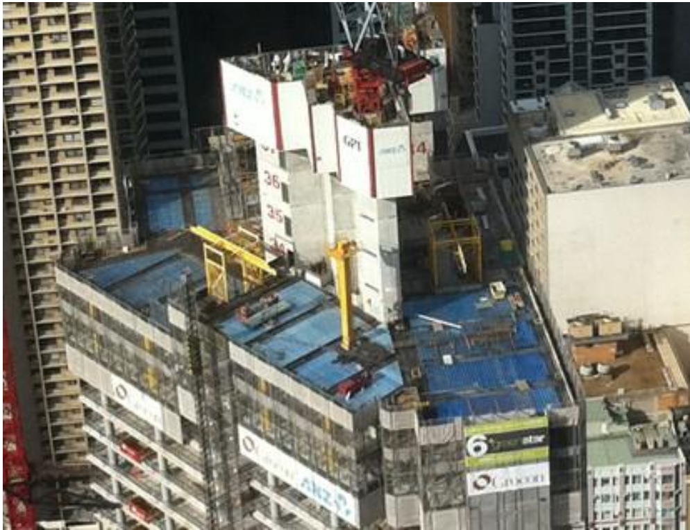
Fig. 4 – Post-tensioned composite slabs
