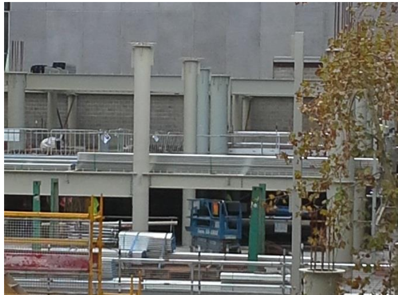
(b) Building during construction
