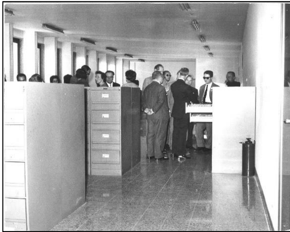
Figure 6.5 Rizzoli Documentation Centre in 1963-1964, CdRcs.
