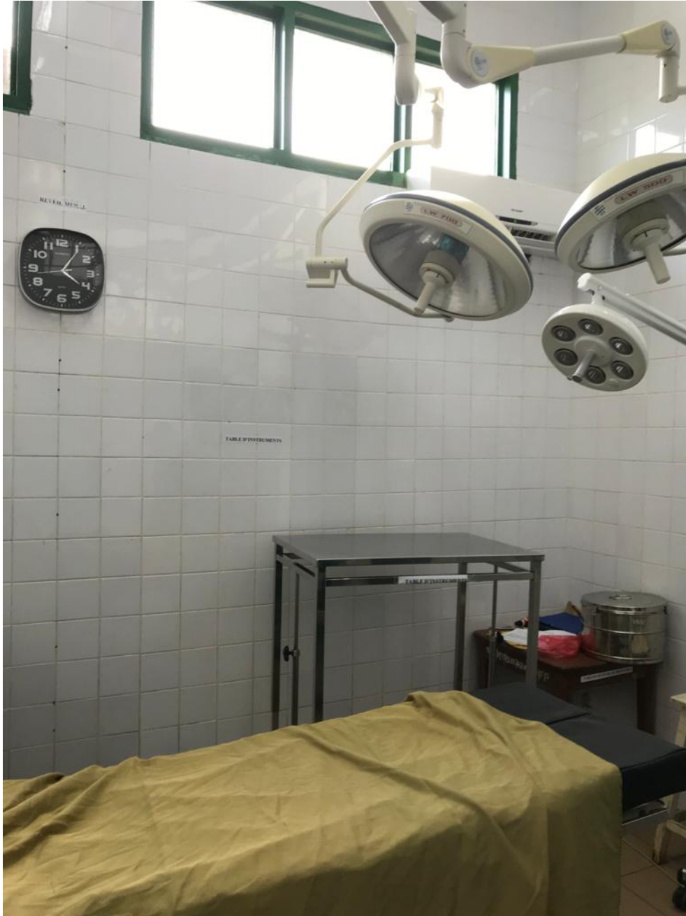
Figure 3.1: Details of a surgical room in CHU d'Abomey-Calavi. The windows are neither sealed nor filtered.
