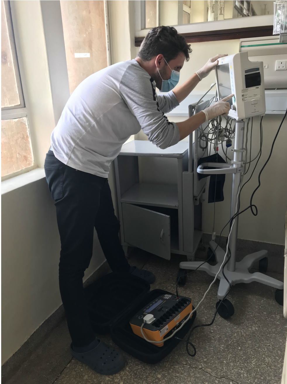
Figure 3.8: Electrical safety measurements
