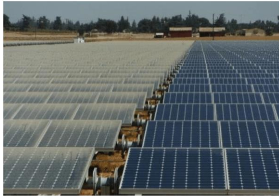
Figure 3-5. Example of soiled 6 panels (left) and unsoiled panels (right) in a large PV power plant [132]
