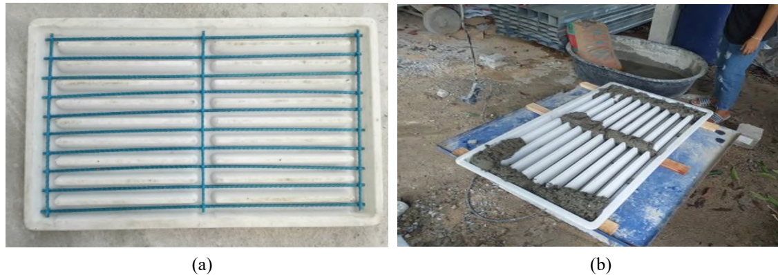
Fig. 4. (a) Plan view of typical slab moulds and FRP bars, and (b) compaction of concrete during casting.
