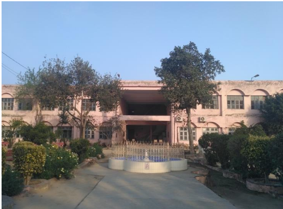
Figure 1.1 Government college building in Haryana
