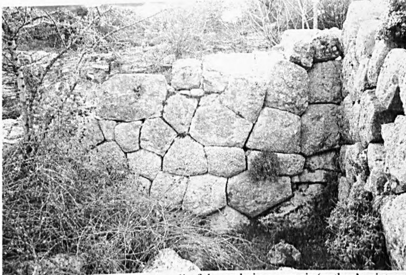
Fig. 39. Ptoion: The polygonal wall of the archaic reservoir (author's picture).
