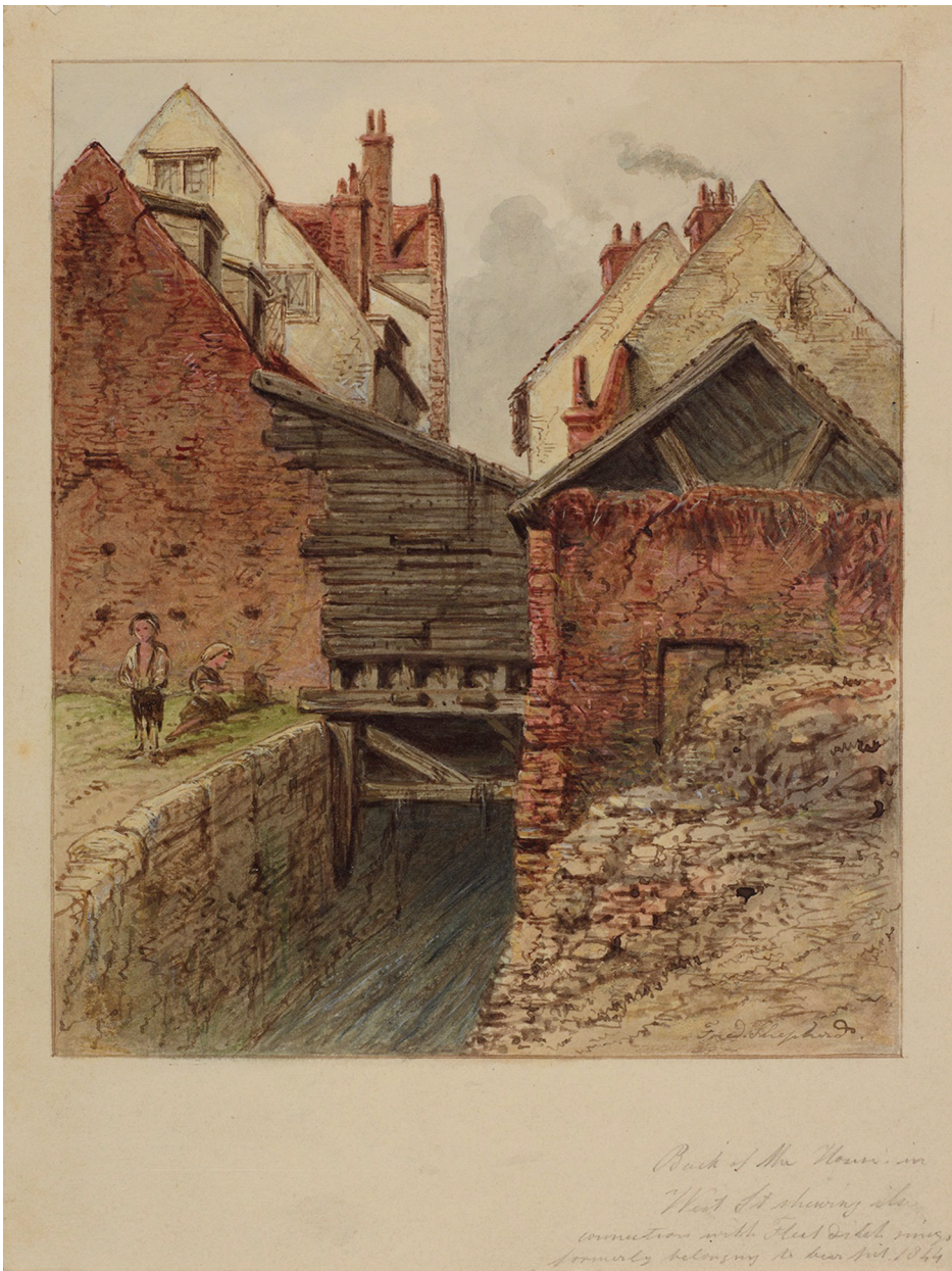
Figure 7. Thomas Hosmer Shepherd, Back of the House in West St showing the connection with Fleet Ditch, c. 1844, © London Metropolitan archives.
