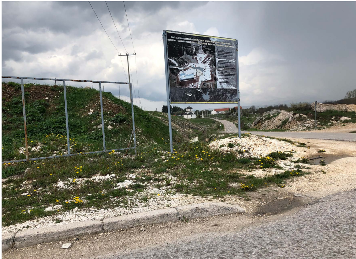
■ A signboard for the construction site for a derivation tunnel for HPP Dabar, the Zalomka near Biograd, the Nevesinjsko Polje, May 2022.
