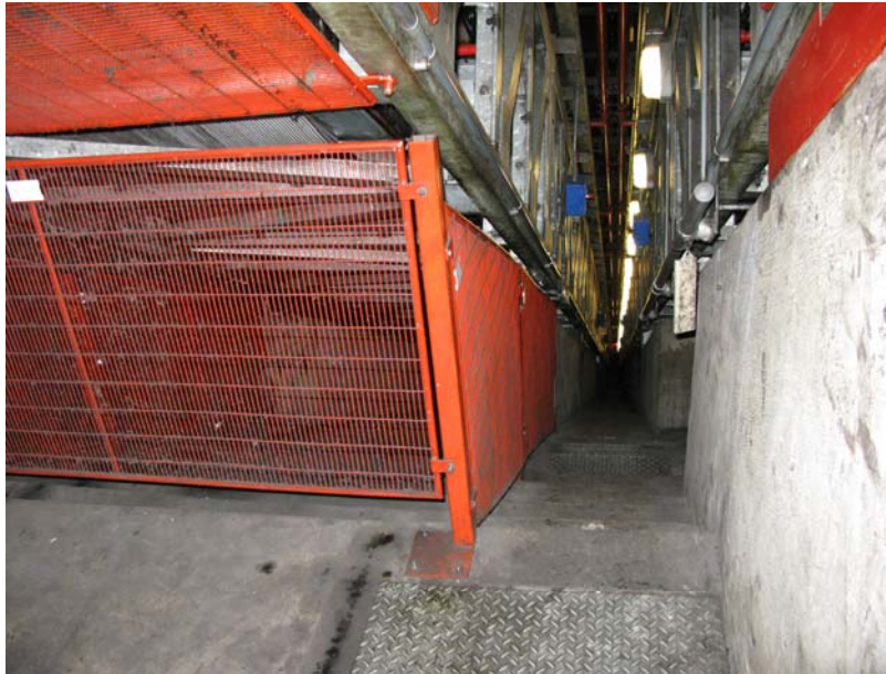
Figure 9. View down the service stairs between escalator trusses.
