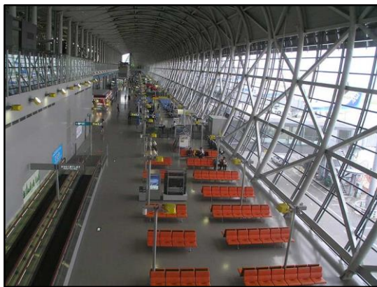
Figure 1.2: Kansai International Airport in Osaka, Japan
