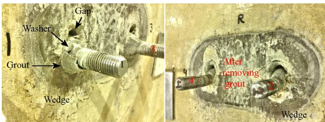
Fig. 6.24. Concrete crushing for FBSC Test 6
