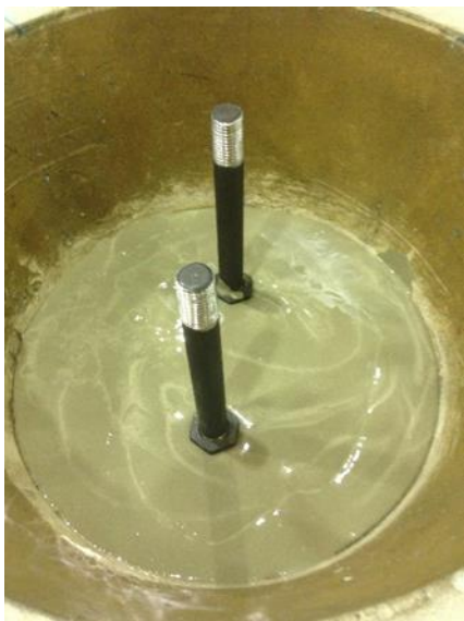
Fig. 4.25. Pouring grout into slab pocket
