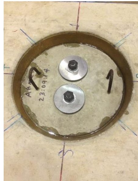
Fig. 4.26. Concrete plug inserted into grouted slab pocket
