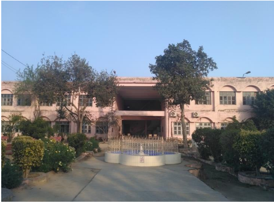
Figure 1.1 Government college building in Haryana
