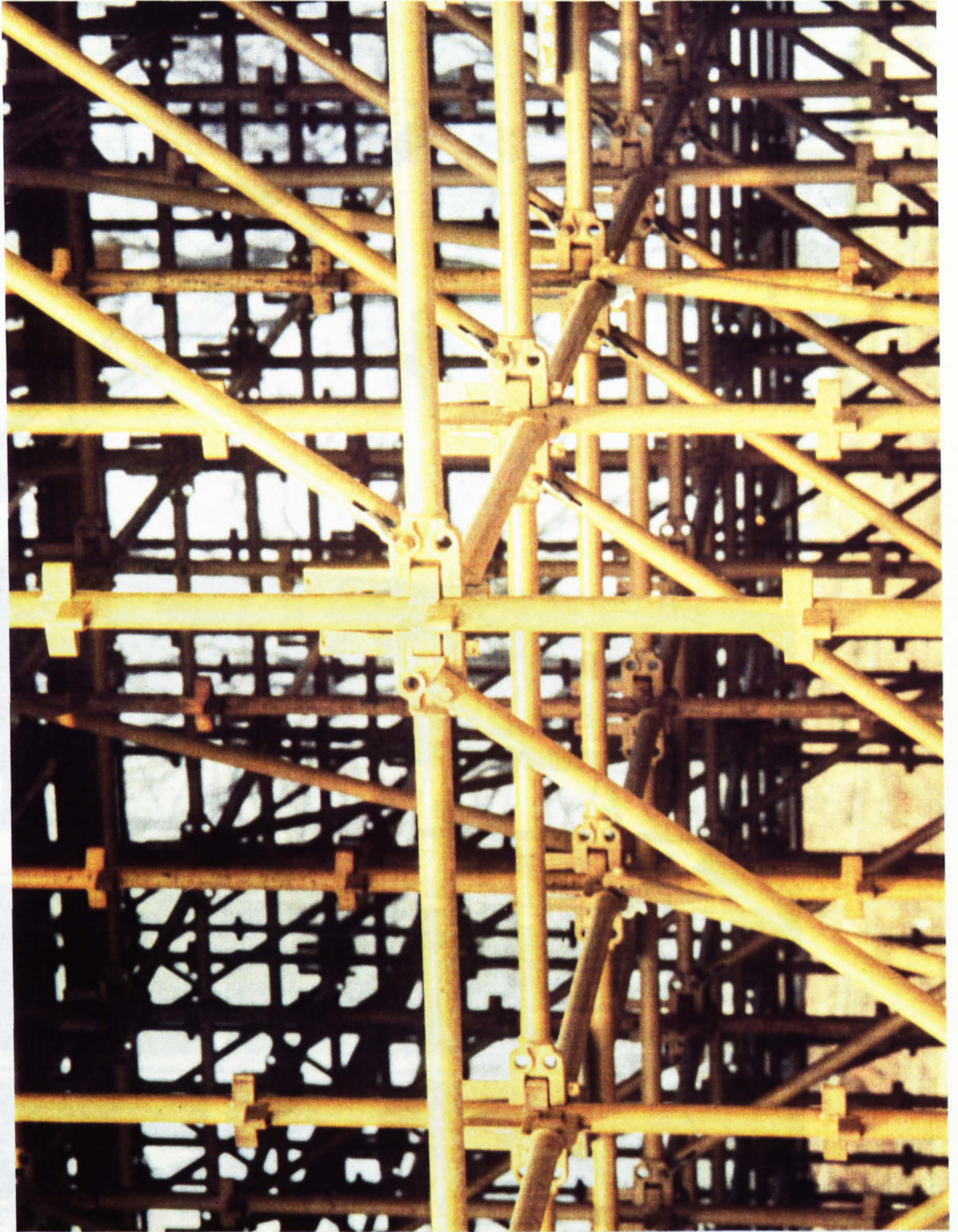
Plate No. 7. View of heavy duty proprietary system showing trigger-brace and coincident node connections.
