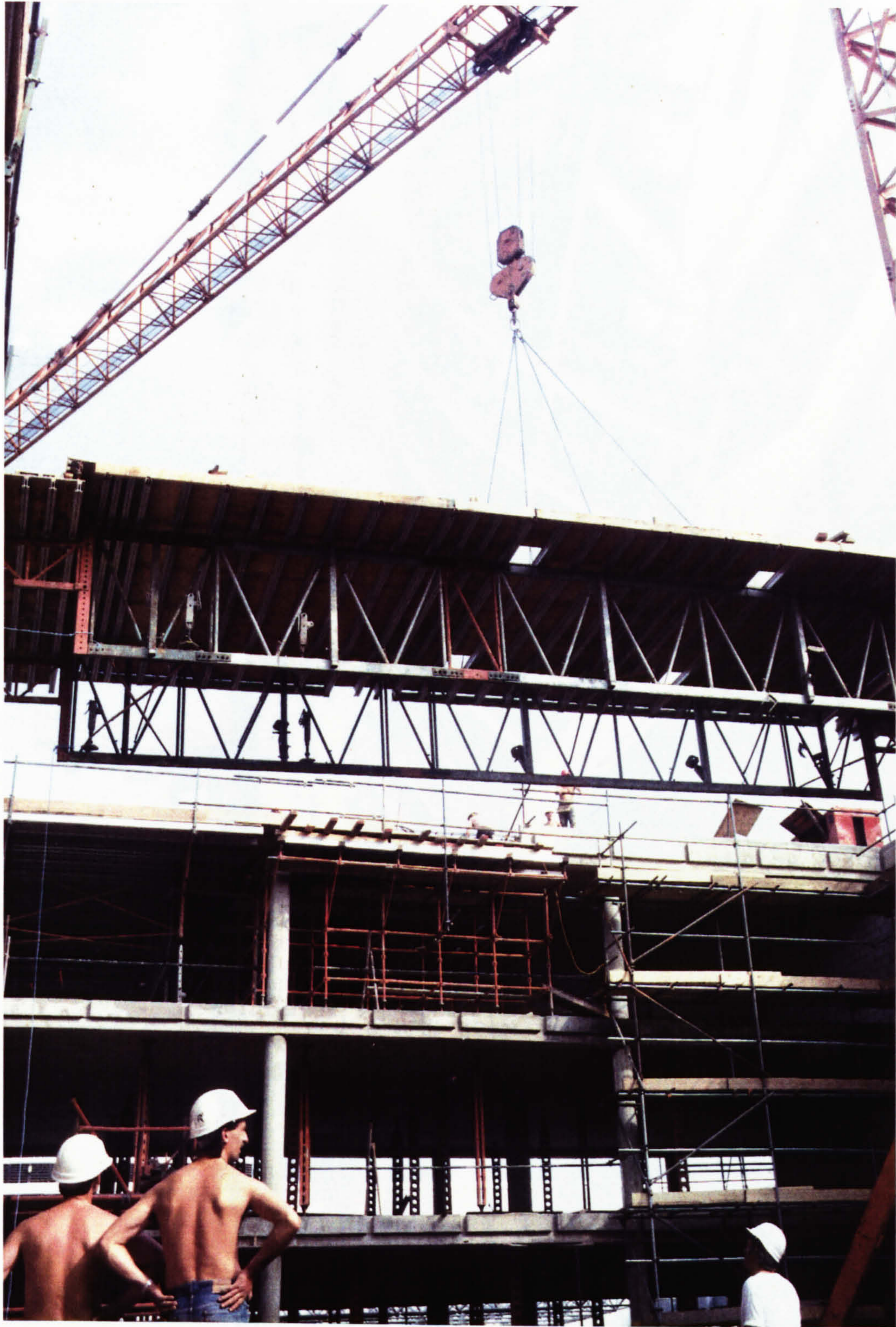
Plate No. 8. Flying form proprietary system and two other support systems.
