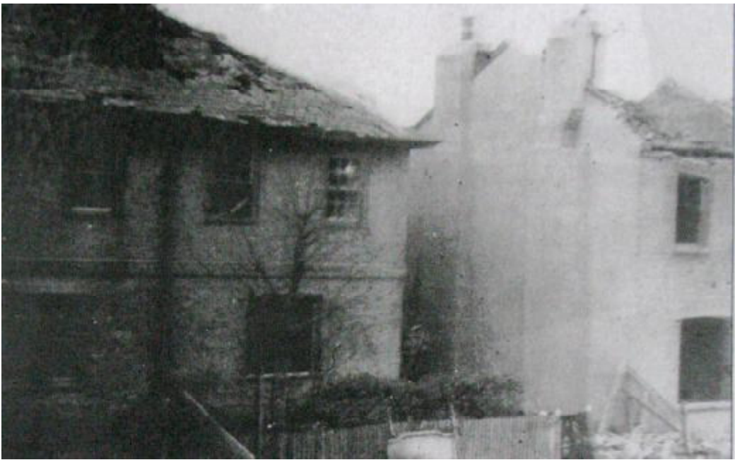
Glengarnock Avenue, Cubitt Town
