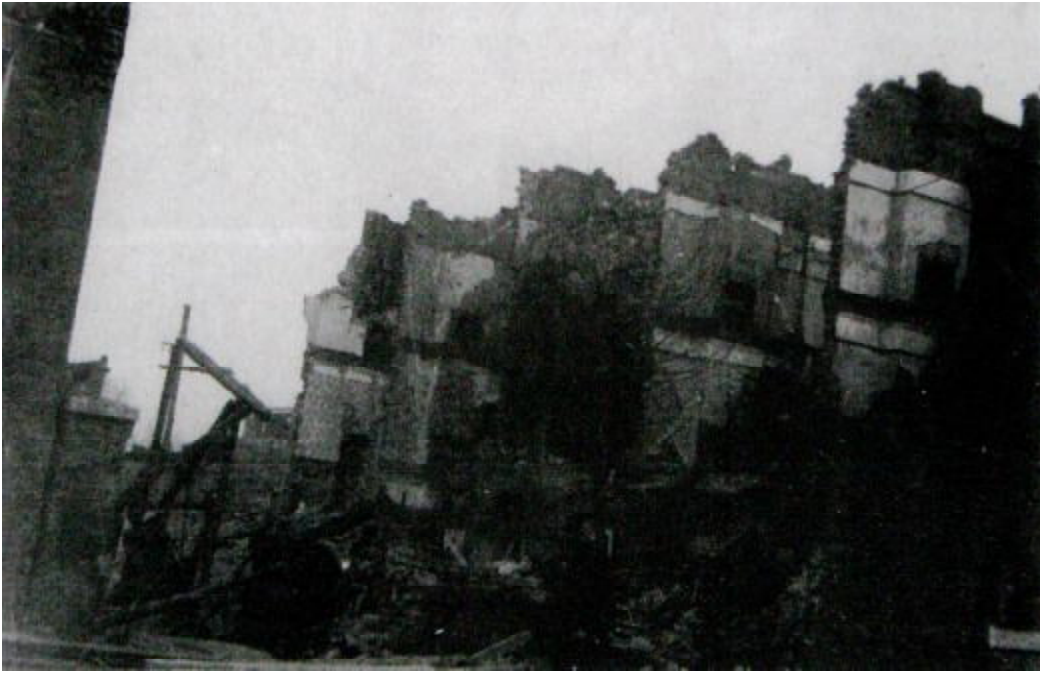
Corner of Parsonage Street and Manchester Road, Cubitt Town.
