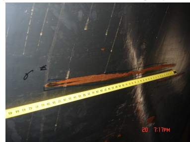
Figure 9 Heated tails observed on the top ring (9F)
