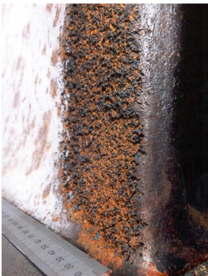
Figure 1.7: Typical sponge-like erosion pattern caused by a leading-edge cavitation attack after 4000 hour operation [6]
