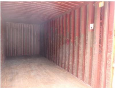
(a) Wall corrugation
